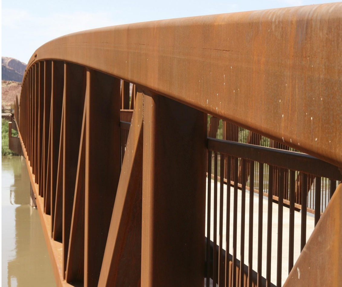
Fig. 21. Application of Cor-Ten steel in bridge construction
