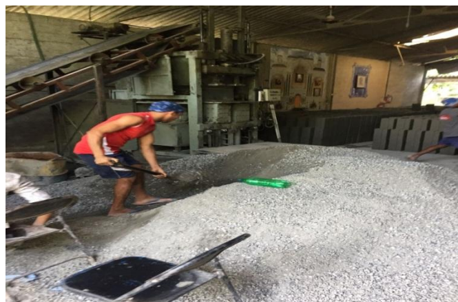
Fig 8 Preparation of cement sand mixture
